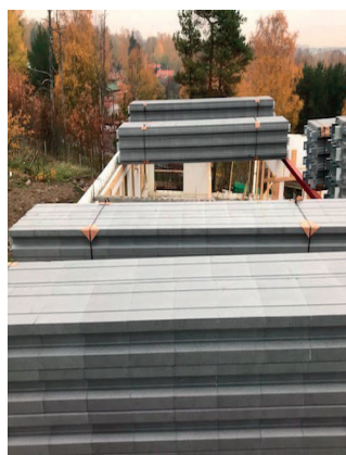
Installation of FKE Elements
